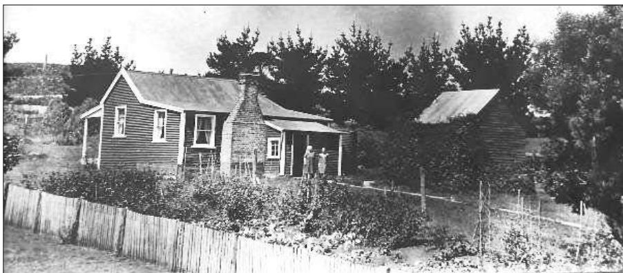
Albertina and Lily Stenberg at the Mawbanna homestead, ‘Sunnyside’. Houses were clad in corrugated iron as protection from the ever-present threat of bushfire.
