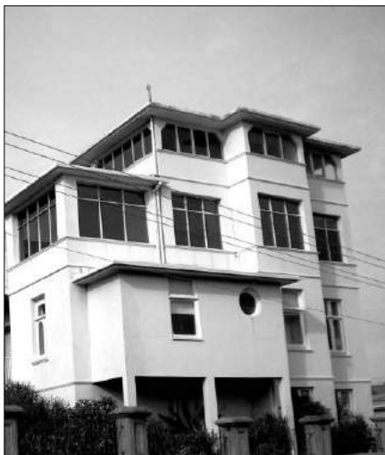
St Margaret's Hospital Frederick Street built for Dr John Ramsay Photograph Jenny Gill
