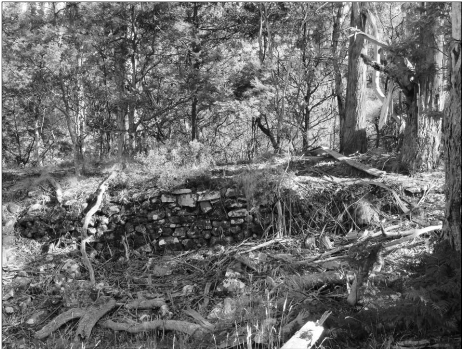
Remains of the dam wall Photograph: Jenny Jacobs
