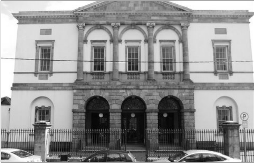
Clonmel Courthouse County Tipperary
