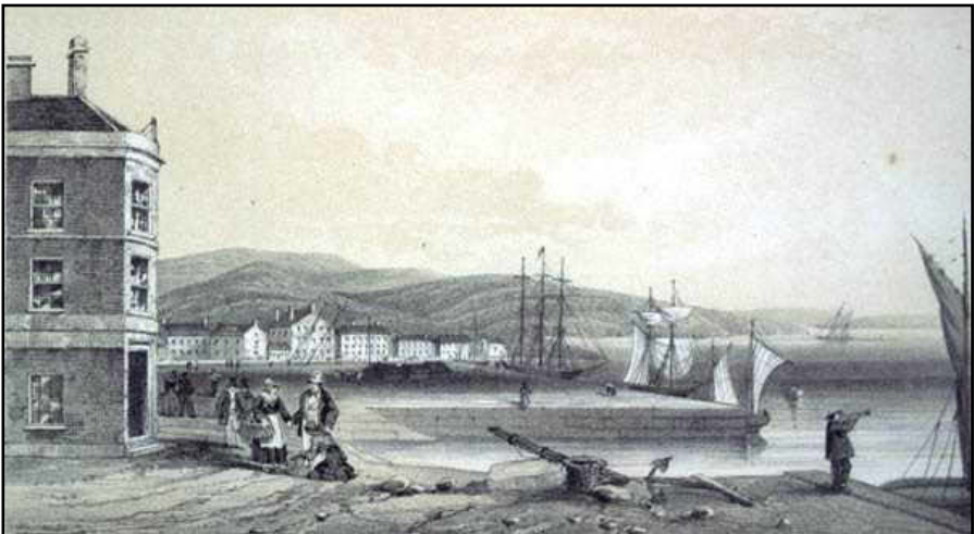
Fig. 2 Alexander McNaughtin owned property on the Old Wharf, 1856.
