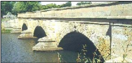
The Historic Ross Bridge
