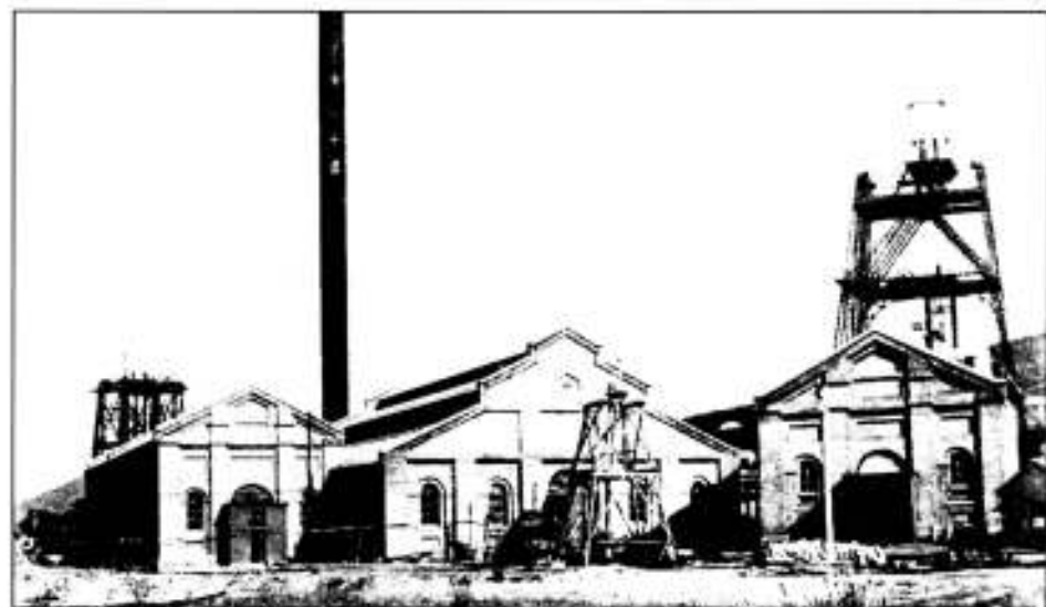
Tasmanian Gold Mining Company site circa 1914. Showing L to R Grub Shaft, Boiler House with Lefroy Headframe in front & Hart Shaft. The chimney stack was 180 ft.
